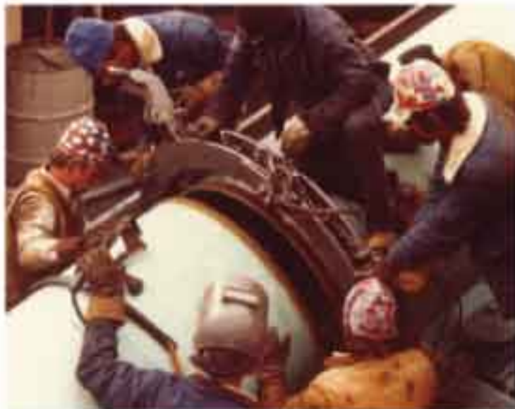
The Jackar can rotate out of position for alignment, welding and grinding without removal of the clamp.
