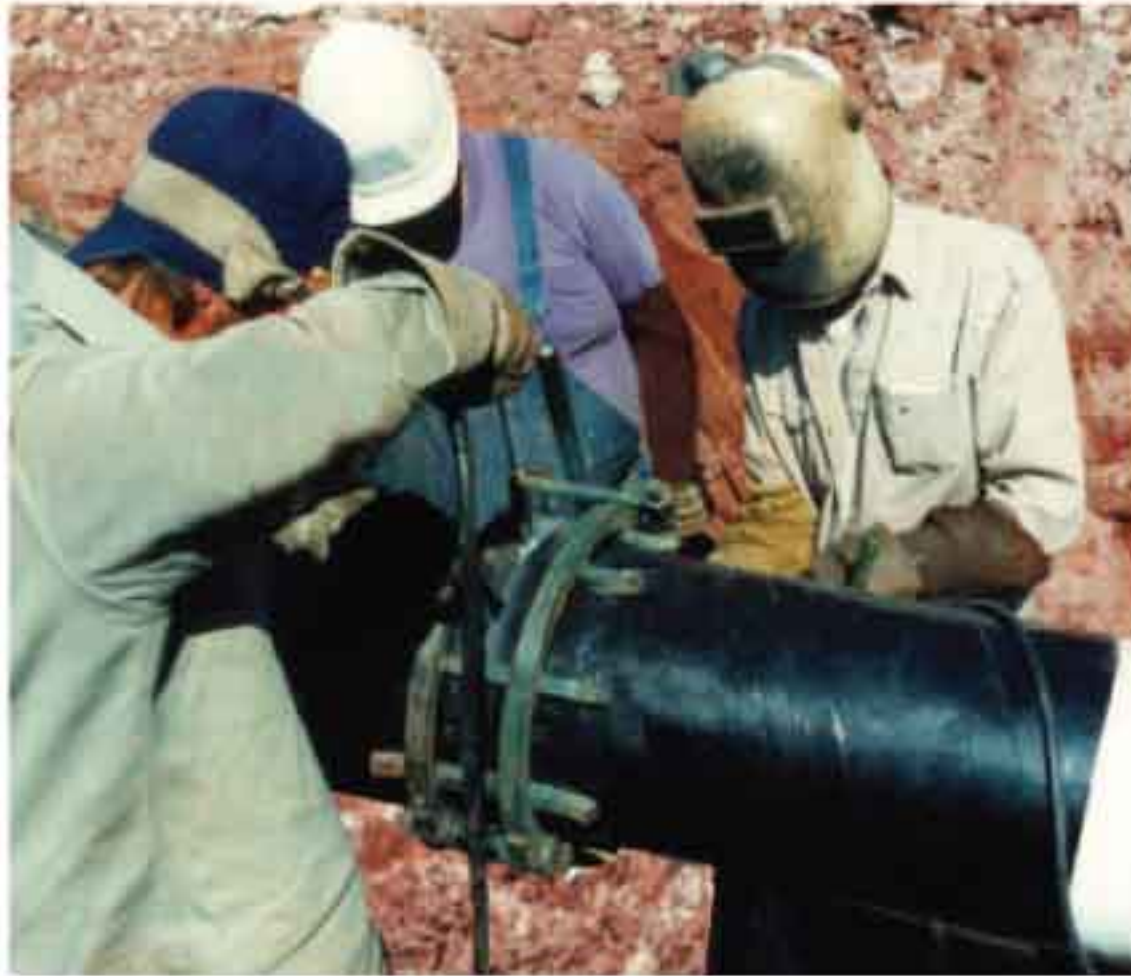
Rapid alignment can be achieved with the Hand Lever Cage Clamp. A Clamp is needed for each pipe size to be aligned.
